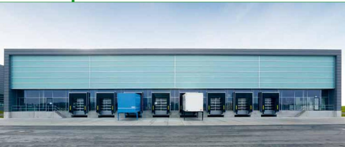
Aluminium and fibreglass, utilised in VARIOPLANplus, are rigid, lightweight materials which make it possible to achieve self-supporting elements without disturbing supporting constructions.
